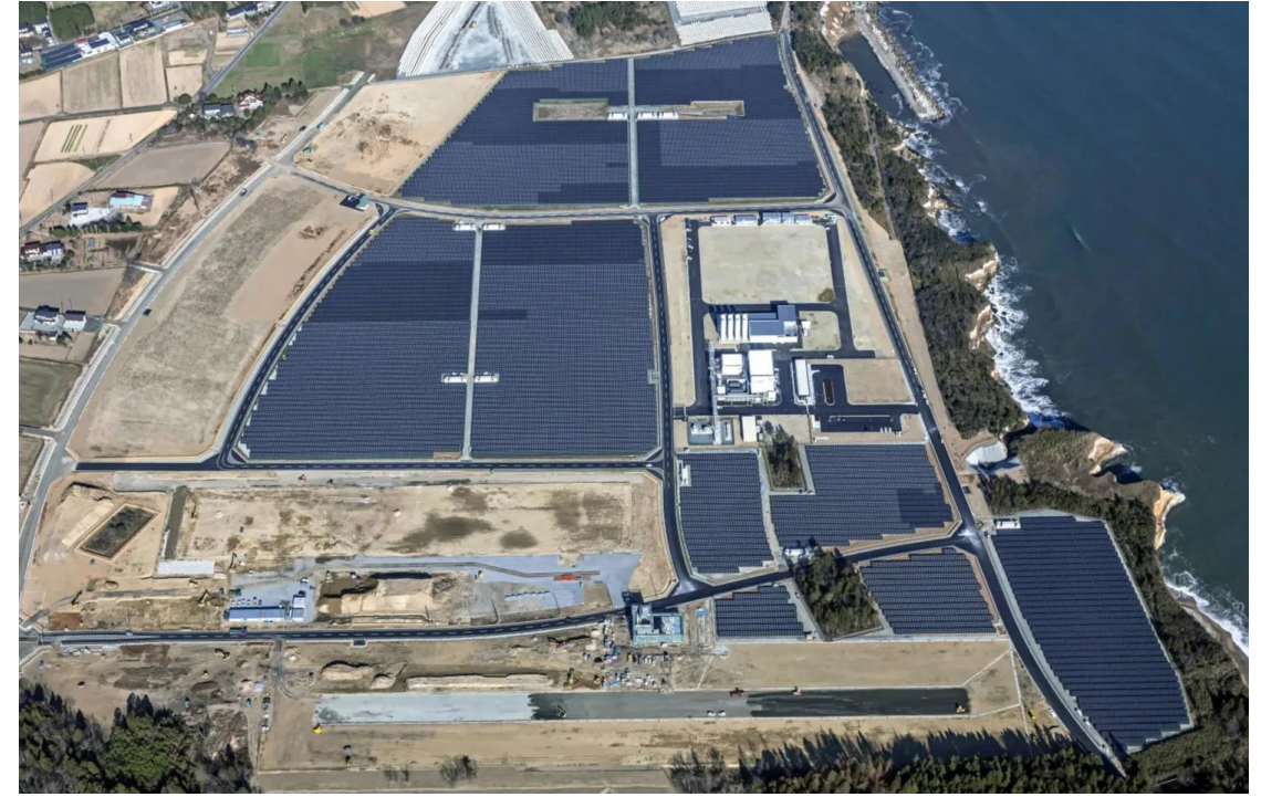
Fukushima Hydrogen Energy Research Field Production Facility (18 ha, 2,500 kgs/day, US $189M)
