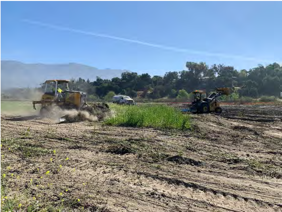
Log Entry Photo D
