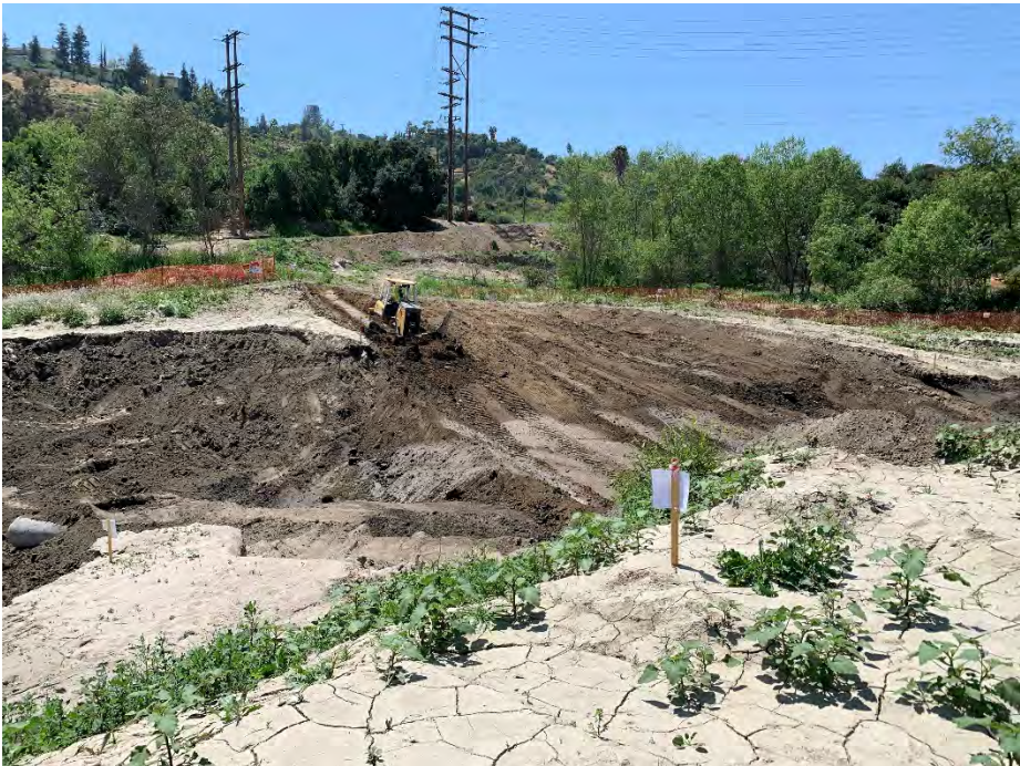
Log Entry Photo D
