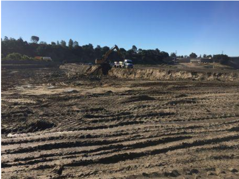
Log Entry Photo D
