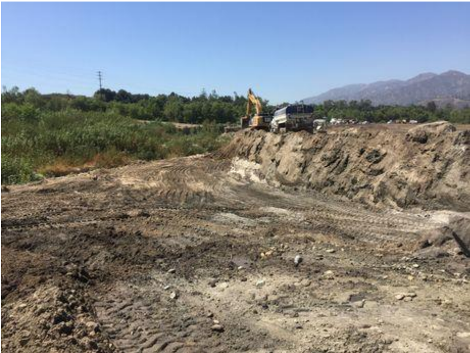
Log Entry Photo D
