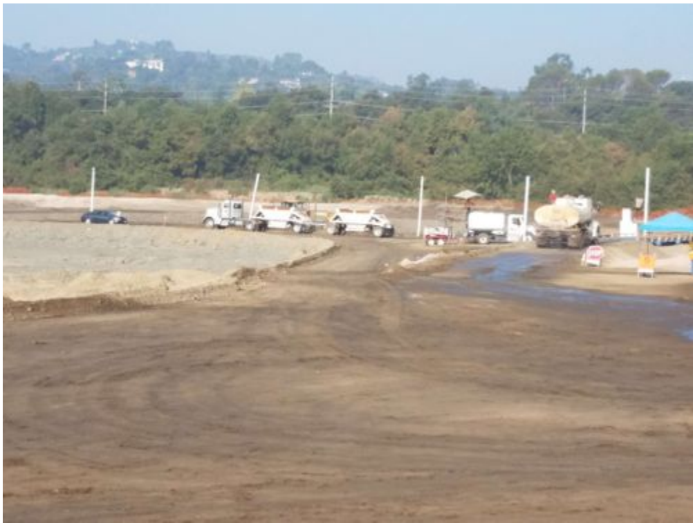
photo_2-20200921_sediment removal_facing W.jpg -118.17348 34.1888
