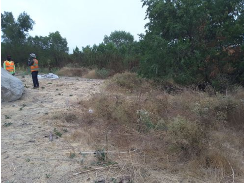
Photo 1-before_clearing edge of DG-4A_ facing N.jpg -118.17511 34.19095
