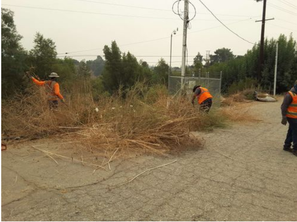
Weed control in process_facing S.jpg -118.17769 34.18701
