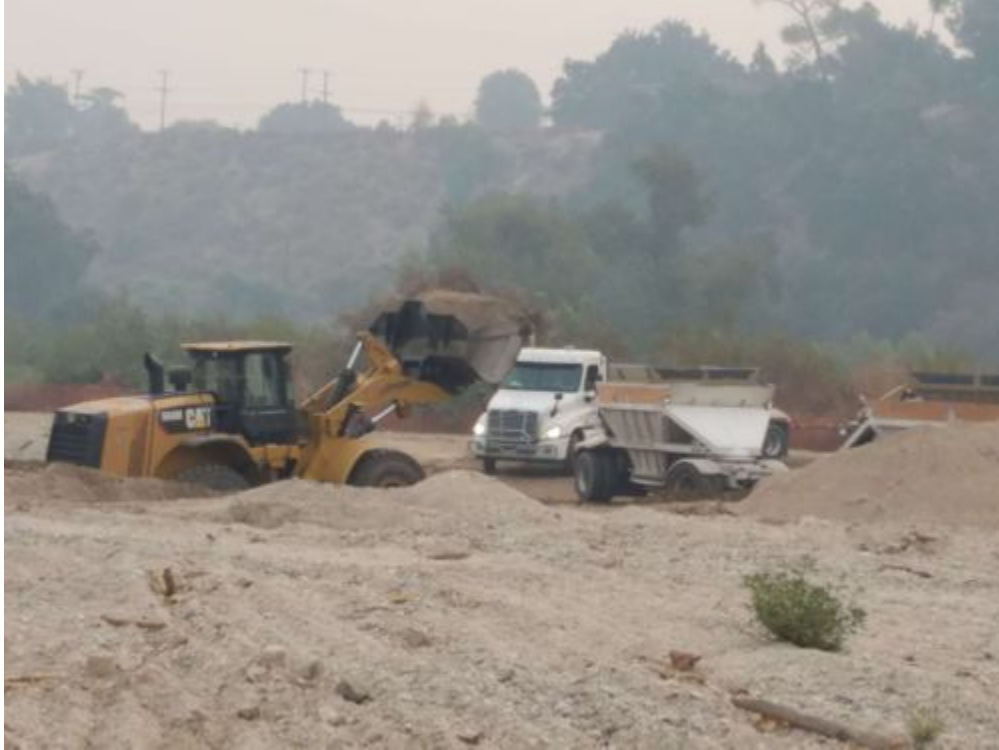
photo_3-20200915_sediment removal_facing NE.jpg -118.17336 34.19169
