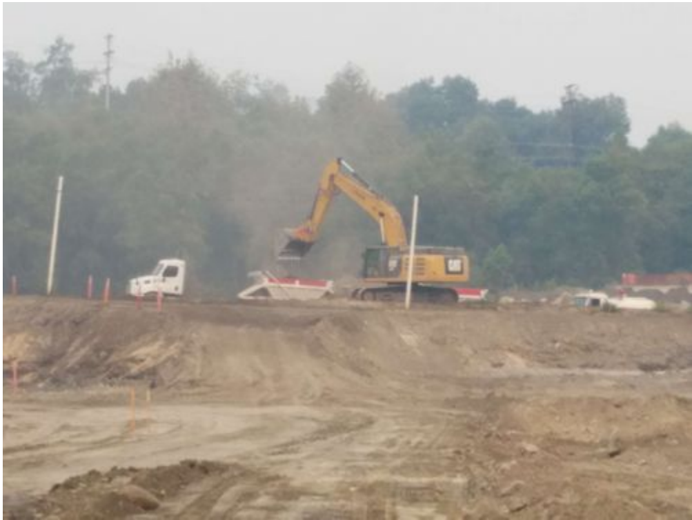
photo_2-20200915_sediment removal_facing W.jpg -118.17411 34.18713
