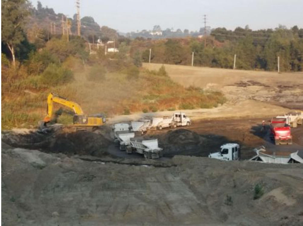
photo_1-20200918_sediment removal_facing W.jpg -118.17437 34.18601
