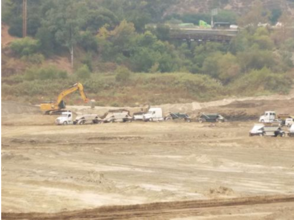
photo_3-sediment removal_facing SW.jpg -118.17322 34.18832
